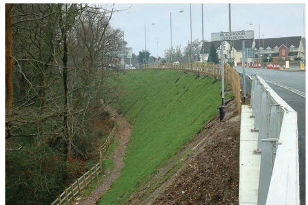
TensarTech™ NaturalGreen rapidly blends into the surroundings.
