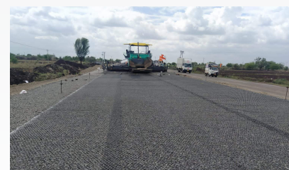
Mechanical stabilisation using multiaxial geogrid on sub-base and wet mix macadam layer on the road section
