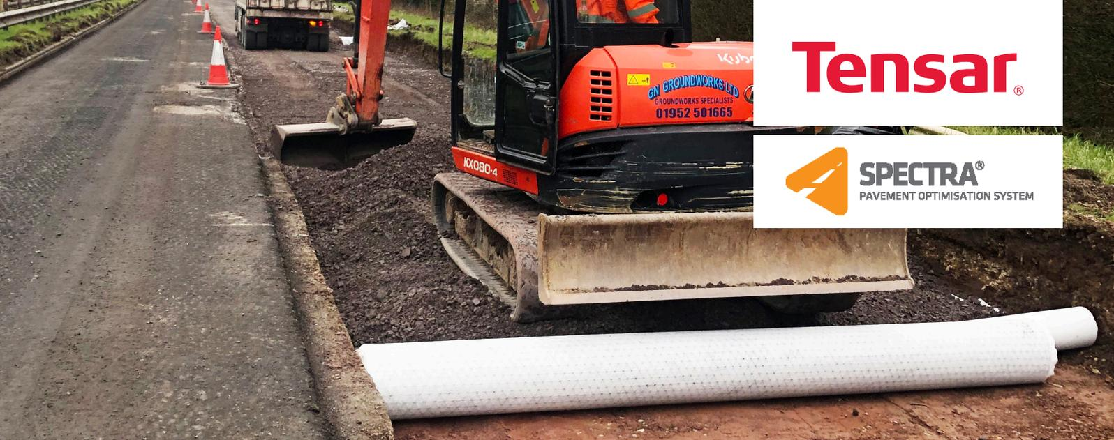
A Tensar geocomposite of stabilisation geogrid backed with a non-woven geotextile was laid in a single layer, stabilising the road's sub-base and offering resistance to upwards migration of fines due to groundwater conditions
