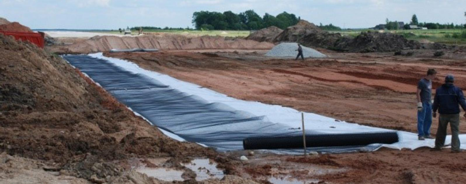
The TriAx geogrid was incorporated into a granular mattress beneath the runway pavement structure.
