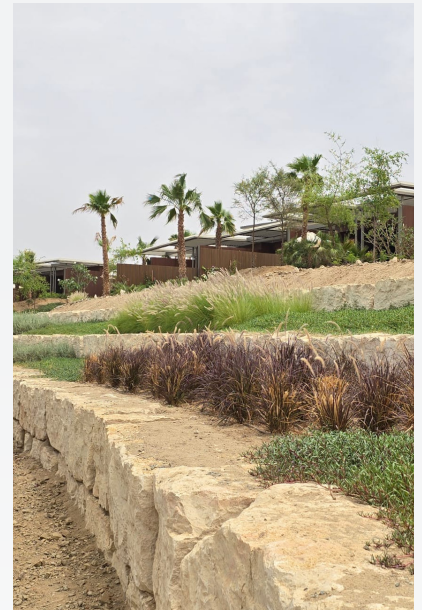
Natural stone boulders and planted vegetation harmoniously blending with the completed Tensar® Wrap Around Facing (WAF) reinforced soil wall system
