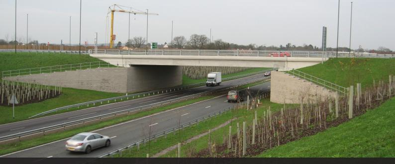
Tensar's TensarTech TW3 retaining wall system was used to build the load bearing abutments and wing walls for the new bridge over the A24.
