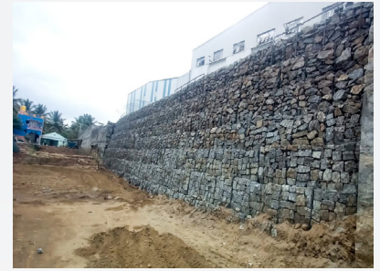
The completed gabion fascia TensarTech® Rock Wall.
