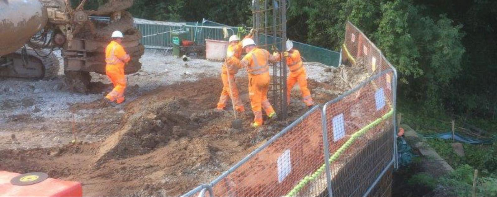
Tensor's TensorTech TR2 temporary reinforced soil wall system delivered a stable, low-cost solution that supported the rig loading of 150kPa, while being quick to build.
