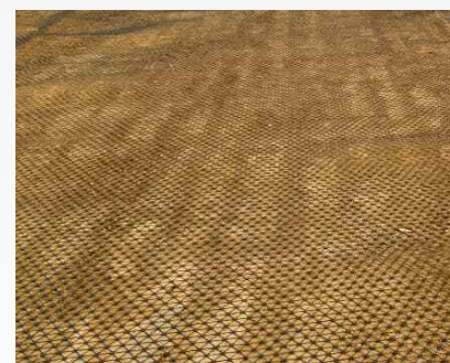
Multiaxial geogrid used in the MSL for the bridge staging platform
