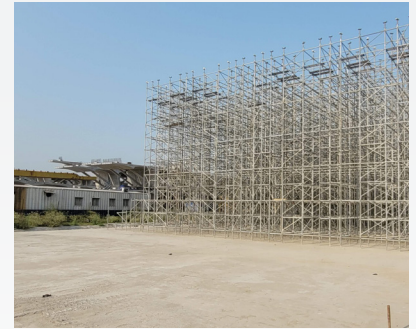
The completed staging assembly of the bridge
