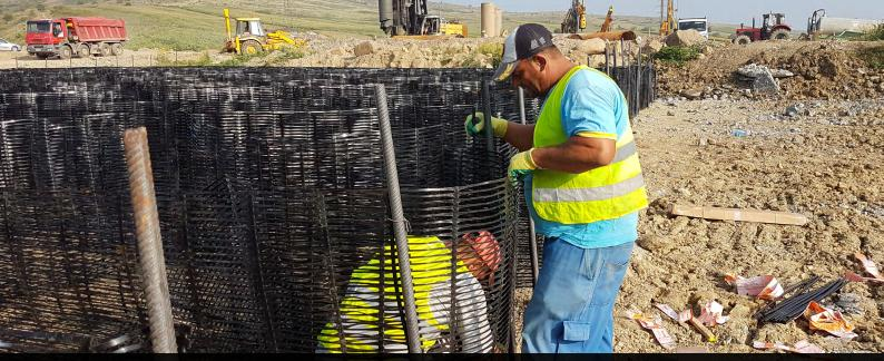
The cellular mattress comprised a Tensar TriAx TX150 geogrid base with Tensar Stratum geogrid cell walls, filled with granular fill to improve bearing capacity and to act as a drainage layer for the embankment.
