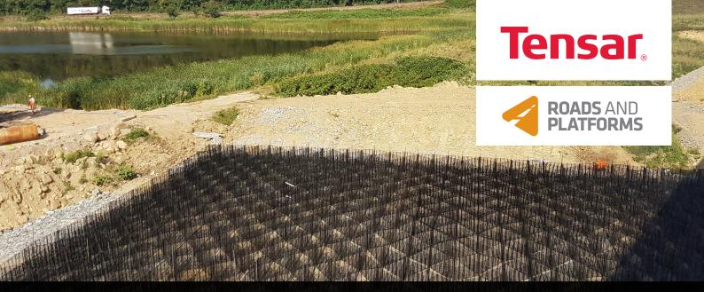
The TensarTech Stratum Cellular Foundation Mattress System formed a stiff foundation for the 300m long embankment carrying the A10 motorway over weak and saturated ground.
