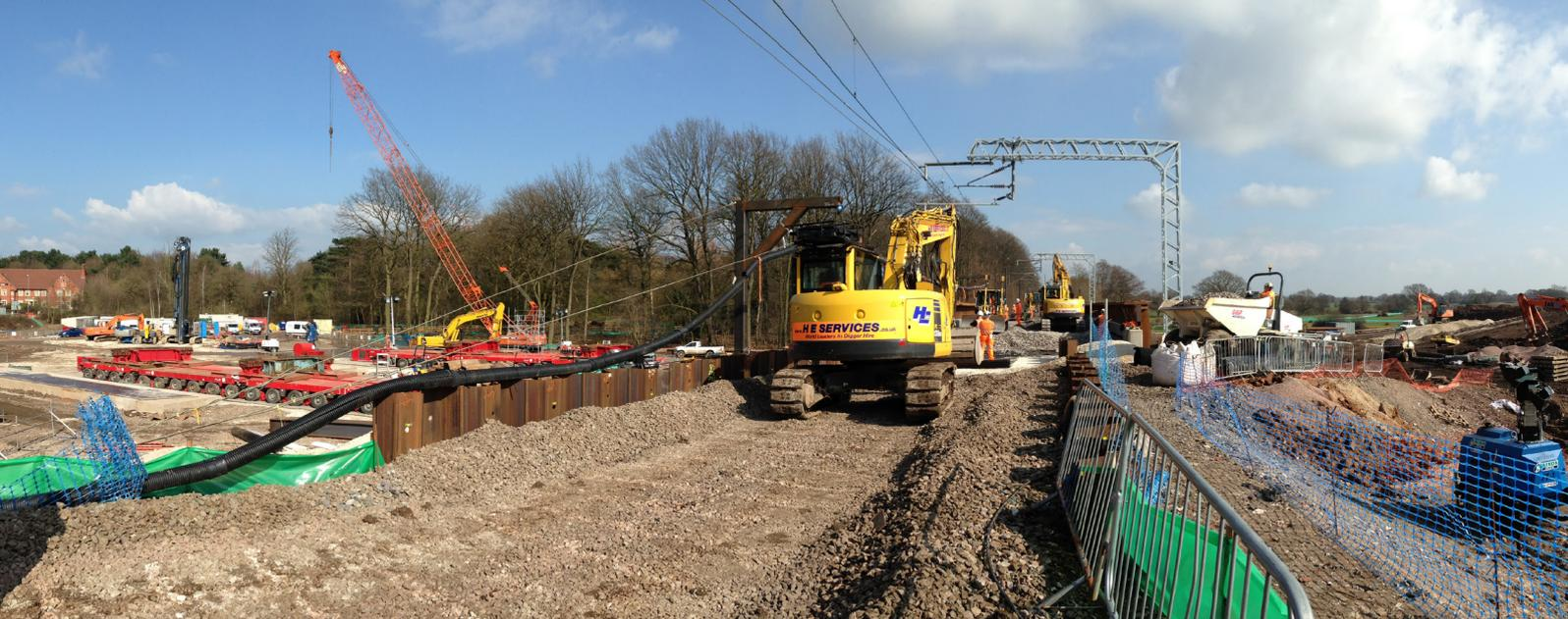
TriAx integrated with unbound track ballast created a mechanically stabilised layer that mitigated overall settlement of the track and differential settlement in the transition zone where the embankment and the bridge deck met.
