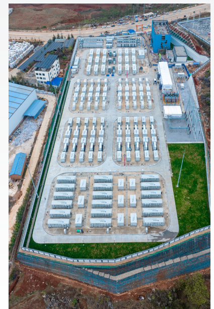
Aerial view of the project
