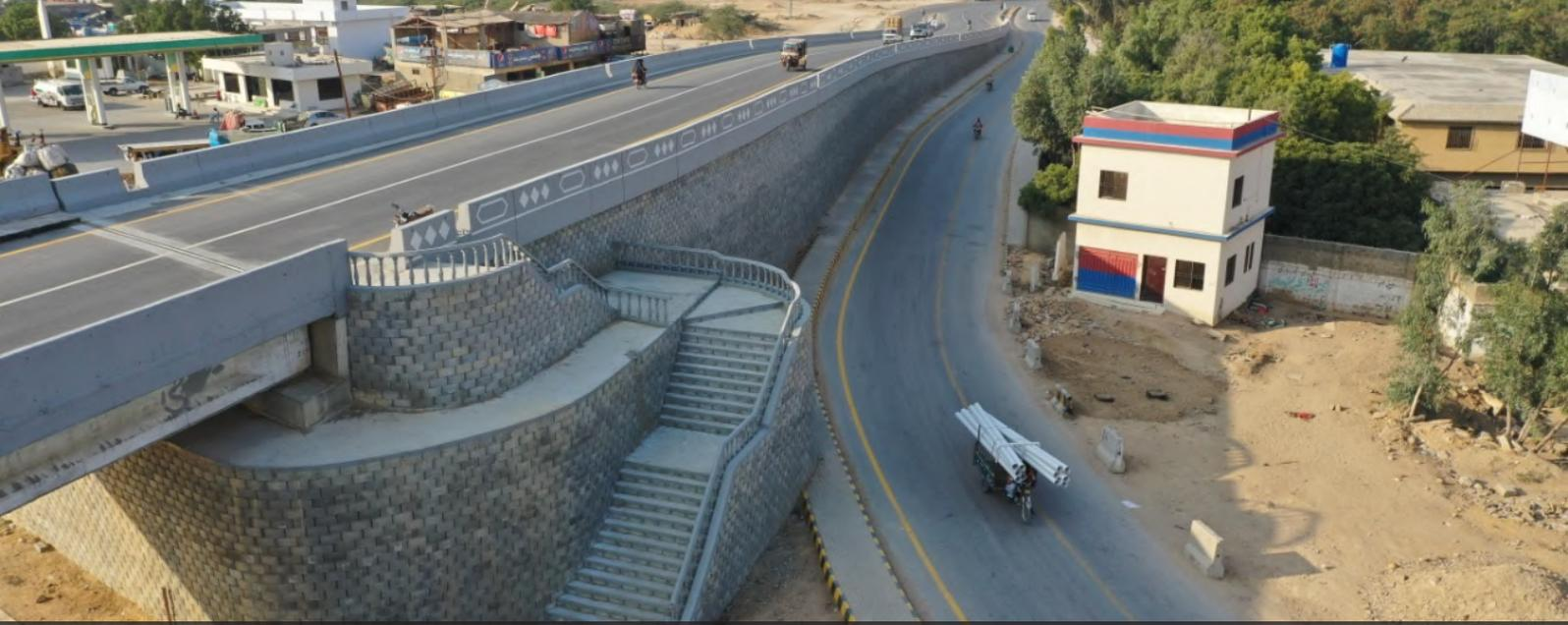
Modular concrete blocks were installed to form narrow curves around the bridge abutments and pedestrian access
