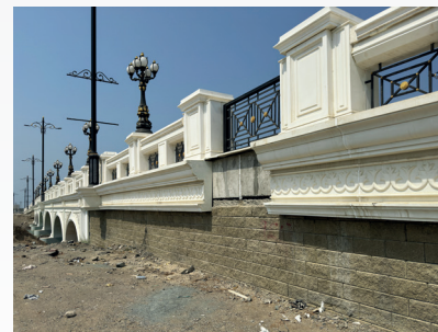
TensarTech® TW1ME supporting the bridge approach embankment.
