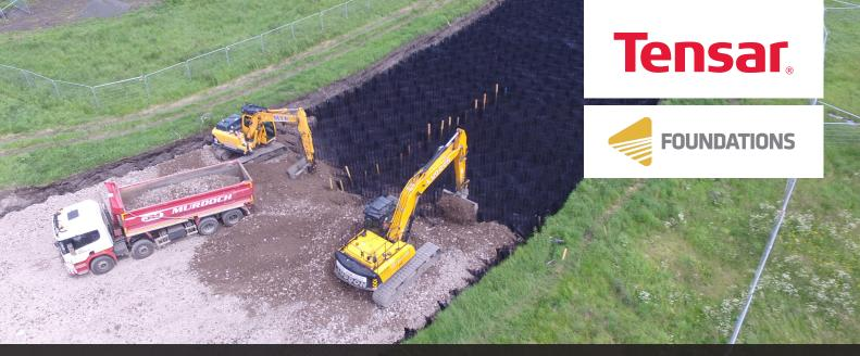
The new link road crosses very weak lake deposits on an embankment supported by a TensarTech® Stratum™ cellular foundation mattress system
