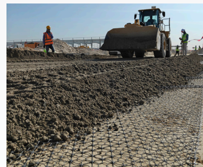
Recycled crushed aggregate base course being placed over HX5.5 geogrid.
