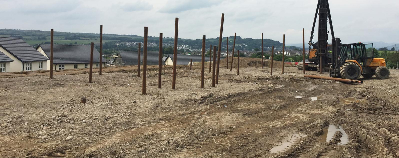
Homes at the upper level had piled foundations, which meant the slope had to also had to be able to support a working platform, formed using TriAx, and piling plant.
