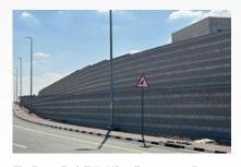
The TensarTech TW1-ME wall system easily accomodates curved and variable height structures
