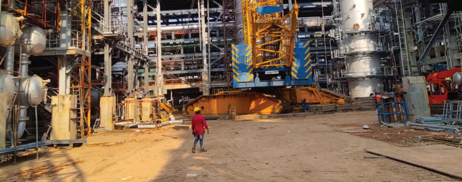
The working platform for the crane lifting refinery components had to support a maximum load of 23t/m<sup>2</sup>, with a maximum allowable settlement of 75mm.
