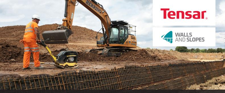
The new embankment was founded on a load transfer platform incorporating Tensar Basetex and a network of driven piles. TensarTech Greenslope created the steep vegetated embankment slopes.
