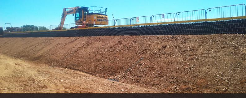
Tensar's TensarTech Greenslope system comprises layers of geogrid that reinforces embankment fill, positively connected to modular, galvanised steel facing units.
