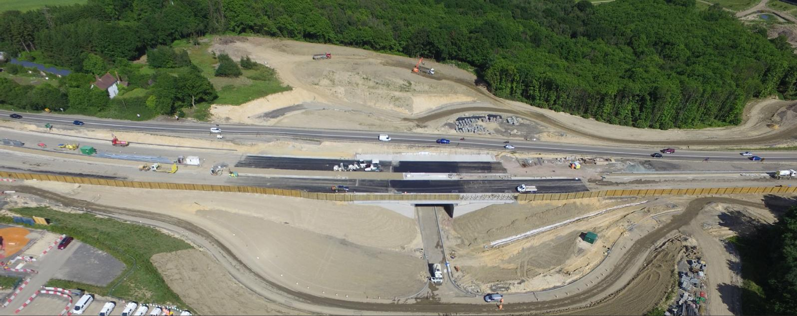
TW3's modularity meant it could be built without heavy lifting equipment or propping, minimising disruption to road users.
