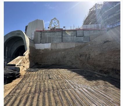
First layer of Tensar uniaxial geogrids being placed over compacted foundation
