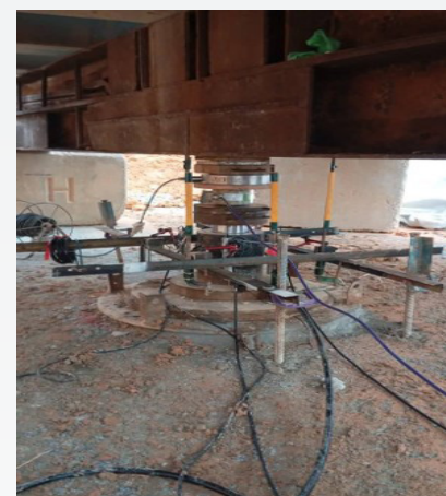
Plate Bearing Test Setup
