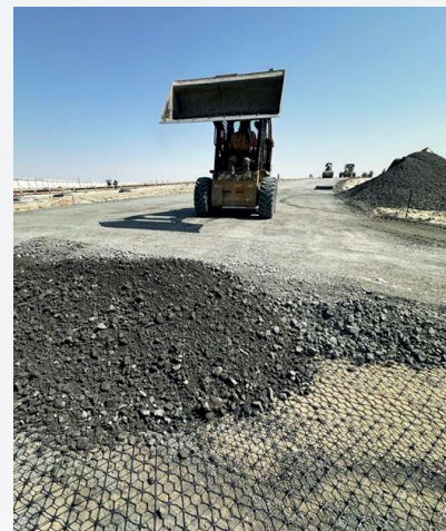
Aggregate base course was spread over the Tensar stabilisation geogrid
