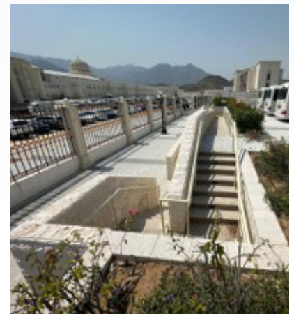
Tiered TW1 MSE Modular Block Wall near Stairs
