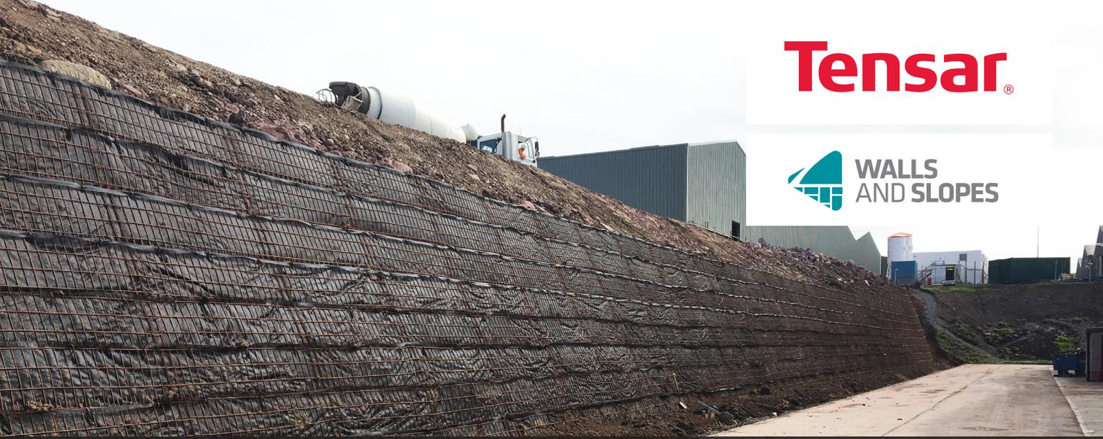
Tensor's TensorTech GreenSlope reinforced soil system helped to maximise development space for new warehouses on the sloping site.
