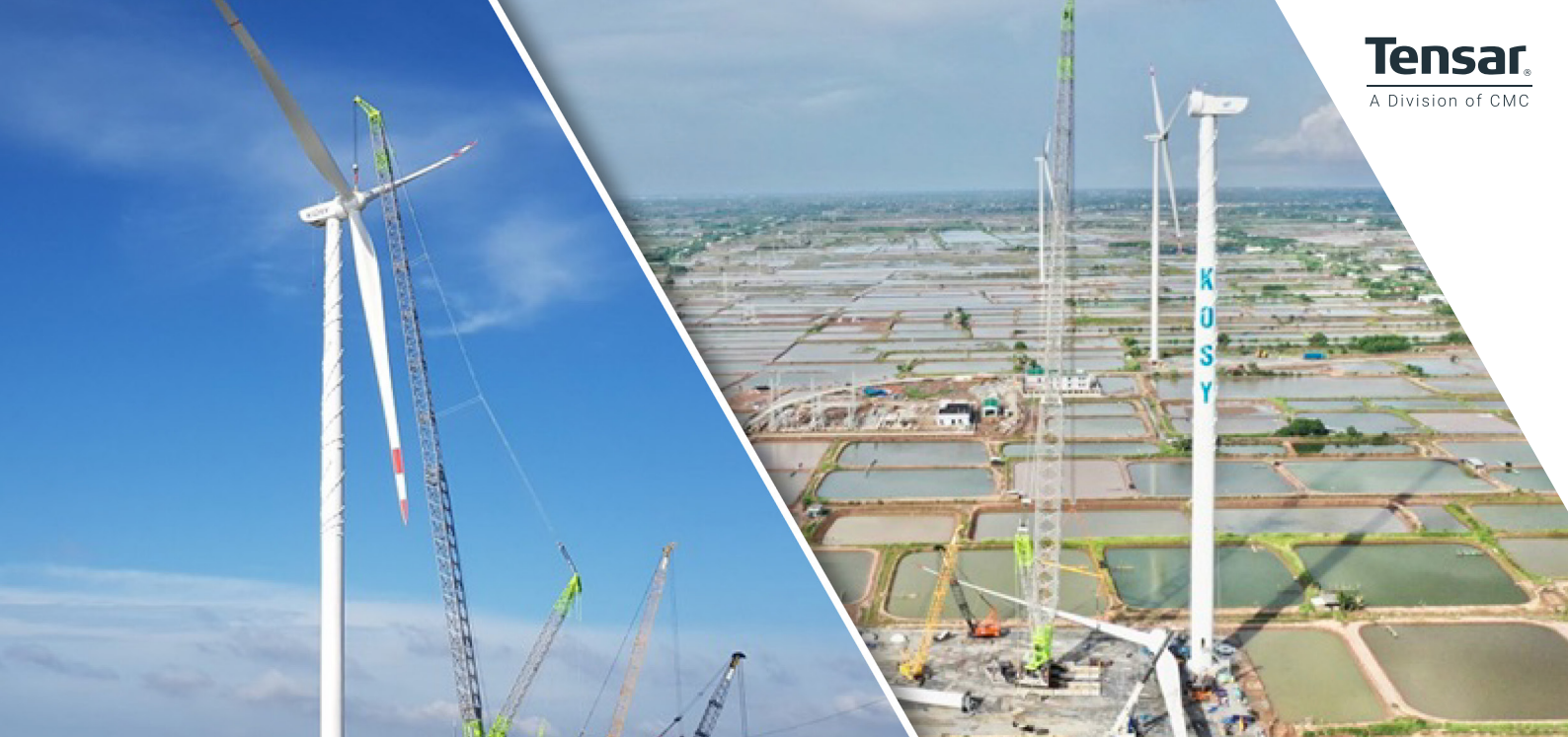
(Left & Right) Zoomlion ZCC9800W crawler crane in operation on the multi Tensar MSL platform
