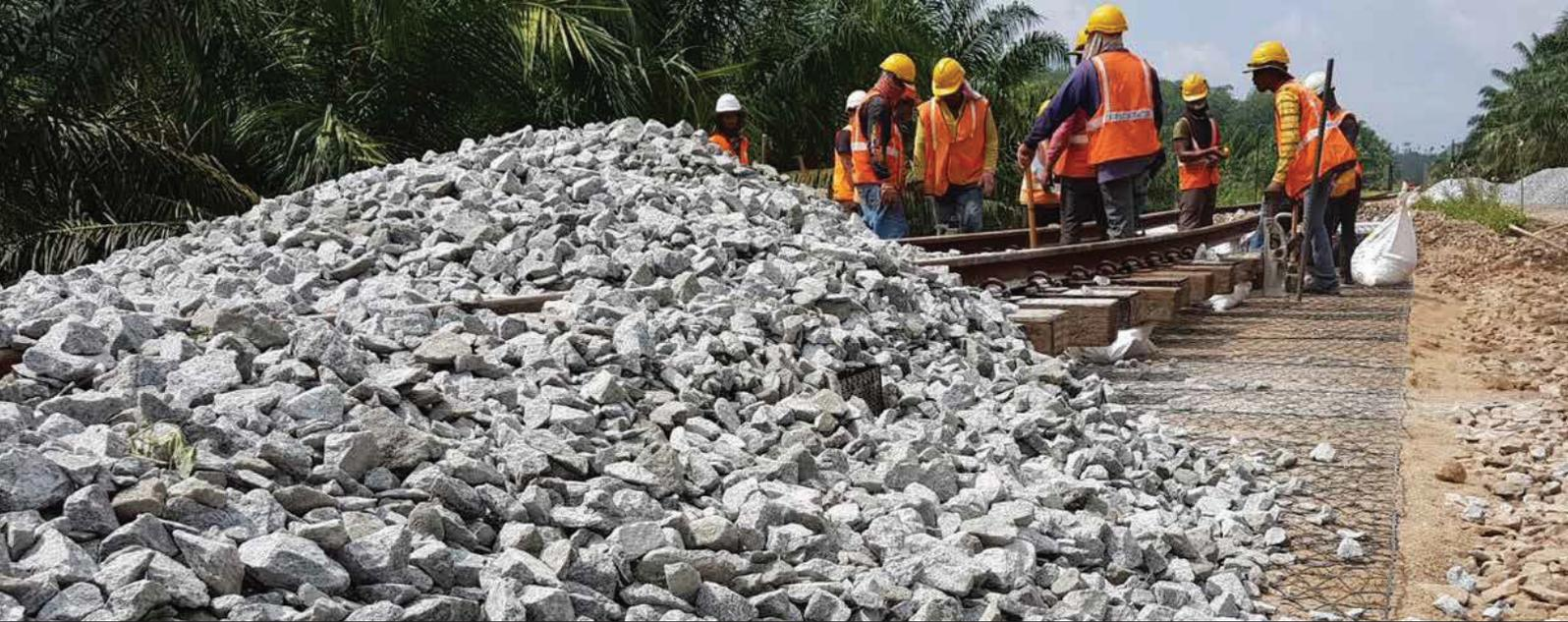
Tensor geogrid helped maintain trafficability of trains at design speed, preventing lateral displacement of ballast and mitigated differential settlement.
