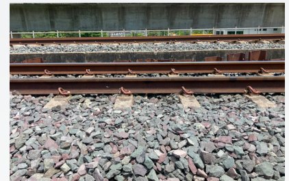
Rail track is supported by mechanically stabilised layer
