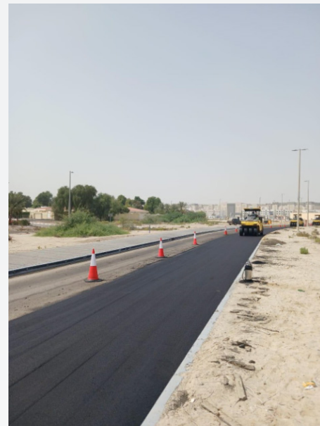
Asphalt overlay undergoes final compaction works over the R60N+C reinforced section.
