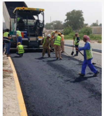
Asphalt paving in progress following R60N+C installation
