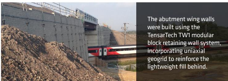
The abutment wing walls were built using the TensarTech TW1 modular block retaining wall system, incorporating uniaxial geogrid to reinforce the lightweight fill behind.
