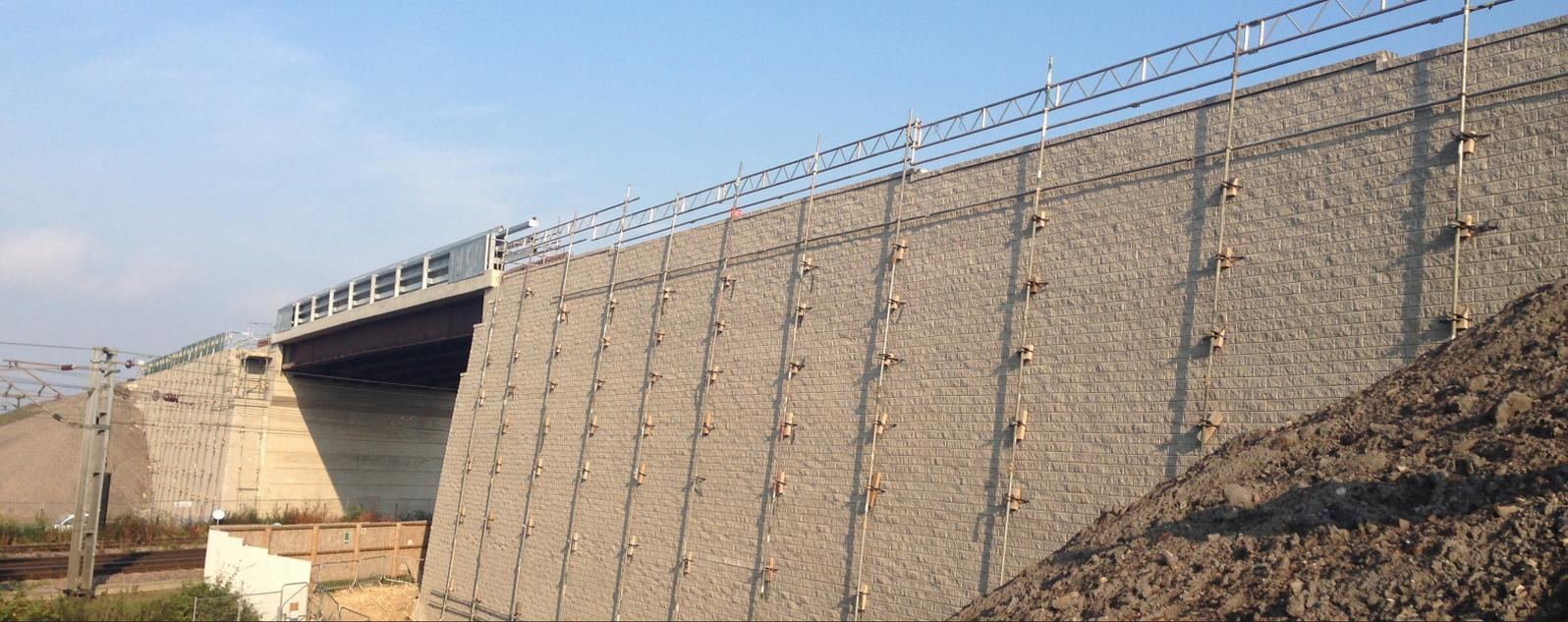
The reinforced earth structures reduced earth pressure behind the bridge abutments, while also reducing the load imposed on the treated ground.
