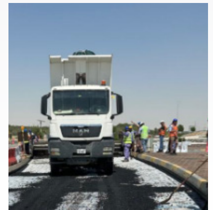
Asphalt chippings evenly spread on glasstex before paving.
