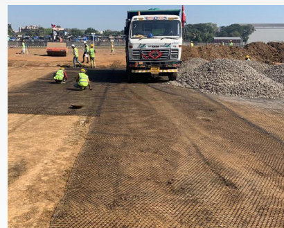
Multiaxial geogrid installation for the graded strip beside the runway
