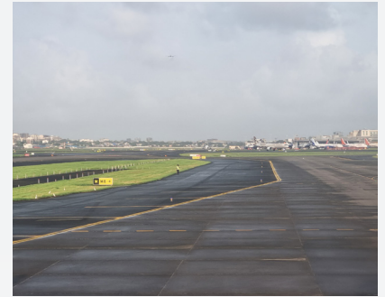
Completed airport runway in 2023.
