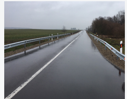
The local road, which was sometimes used by military traffic, had become cracked and damaged due to settlement of the underlying weak clay soils. Photos of the road before and after reconstruction.
