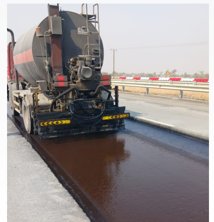
Leveling the soft subgrade prior to laying geogrid.
