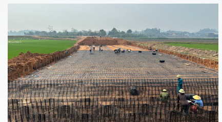
Installation of the TensarTech Stratum Cellular Foundation Mattress for ground improvement solution
