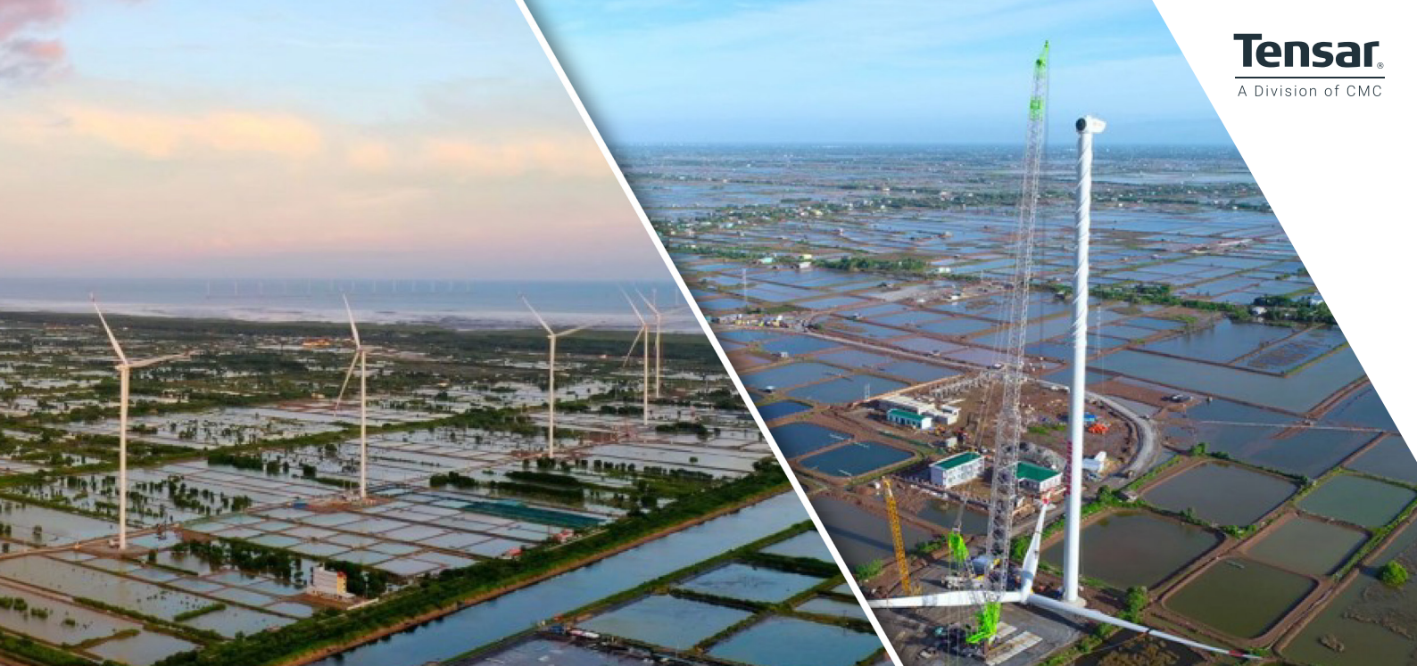
(Left) Completed scene of one project's line/branch in October 2021 | (Right) Zoomlion ZCC9800W crawler crane in operation on a stabilised platform
