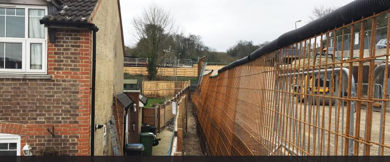
Tensar's TensarTech TR2 reinforced soil retaining wall system enabled the platforms to be built right up against homes and gardens, maximising the safe working area.
