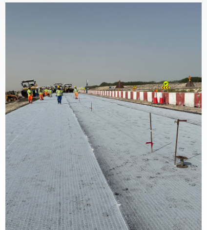
Glasstex R60N+C installed ensuring sufficient overlapping at joints.
