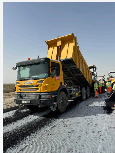
Paving works in progress after curing and bonding of Glasstex R60N+C
