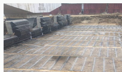
A close up of the installation of ARES Reinforced Soil Wall at Lower Parel Bridge.
