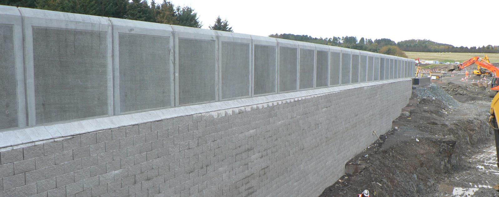
Tensor supplied specially-manufactured 45° chamfered wall caps for additional edge safety.
