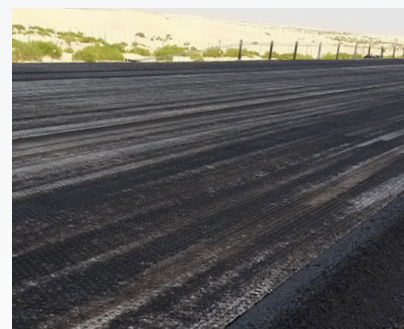
Tensar AX5-GN asphalt interlayer in place prior to overlaying
