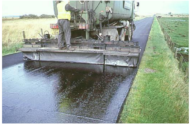
Figure 2: Bond coat application
