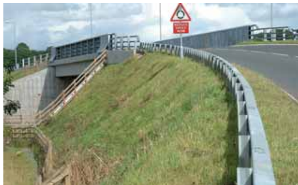
Short construction times contribute to cost savings of up to 75% compared with more conventional solutions and also minimise traffic disruption.
