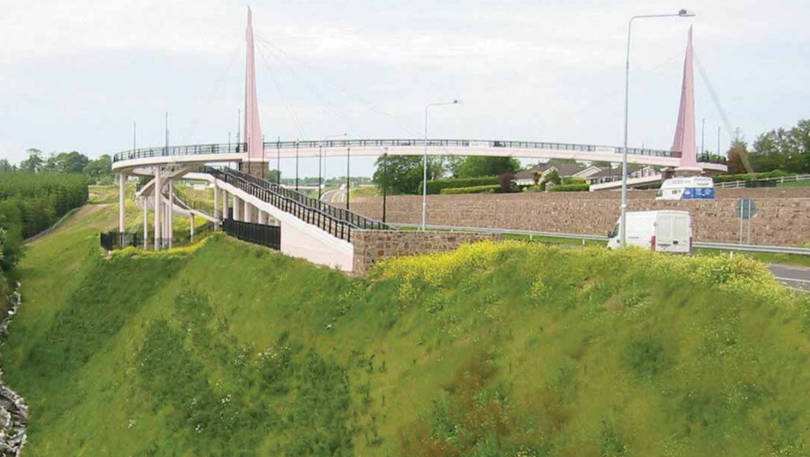
Always keeping one eye on the local environment, Tensar tech NaturalGreen Systems enable you to complete projects with minimal disruption and allow possible use of site-won fill.
