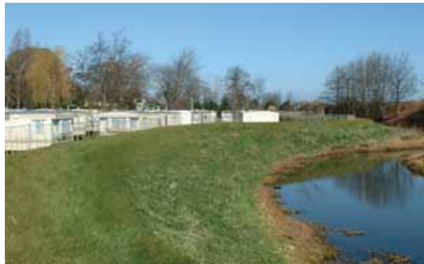
Because Tensar tech NaturalGreen systems minimise off-site disposal of soil and the import of fill, the project's carbon emissions can be significantly reduced.
