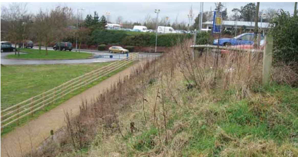
Tensar tech NaturalGreen systems produce a face that is stable and steeper than an unreinforced slope, as well as being naturally attractive.
