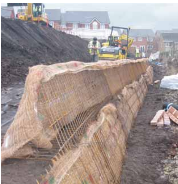
Steel facing units are securely connected to the geogrid reinforcement.
